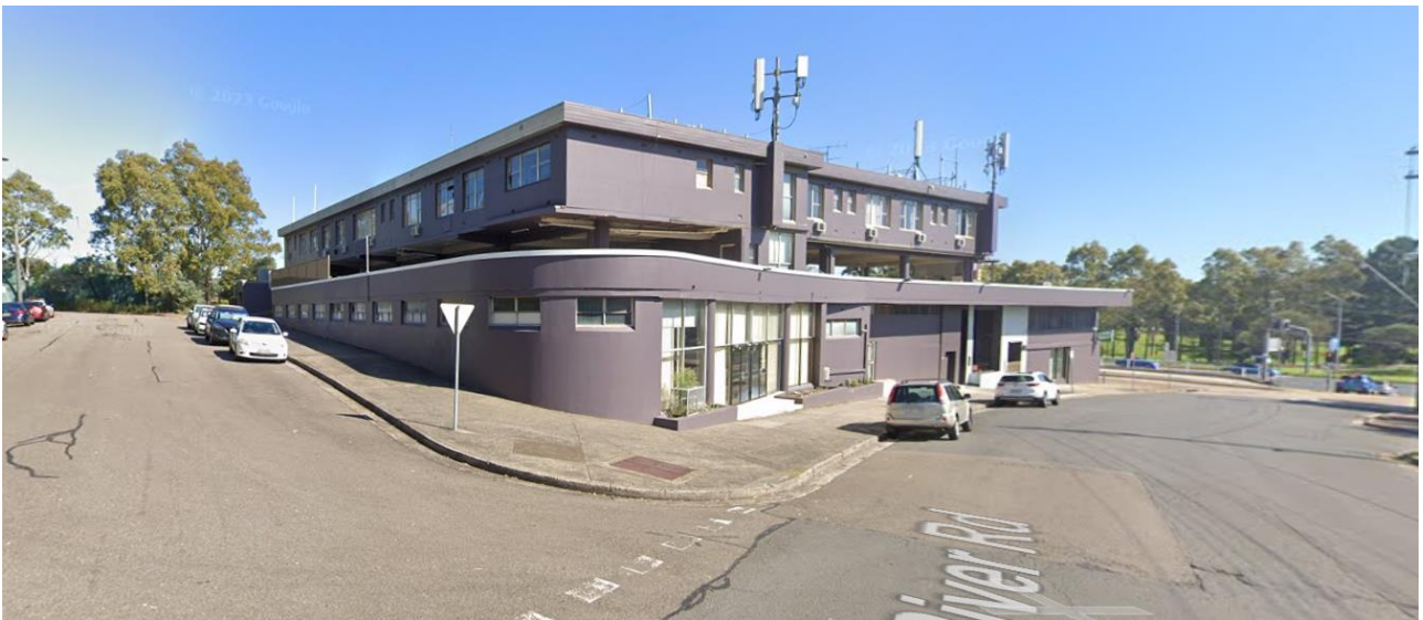
Above: as viewed from the corner of River Road and Lister Ave
